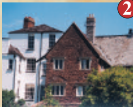
Master's House, Chilcot's School
